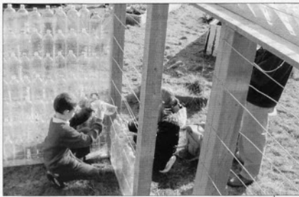
Photo 9: Stacking the Bottle Wall
